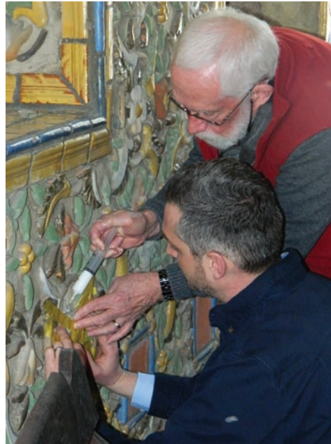
CONSERVATOR ANDREW FEARON works with Fonthill volunteer Hugh Downing to demonstrate the proper technique for injecting adhesive behind loose and endangered tiles in the Breakfast Room at Fonthill.
