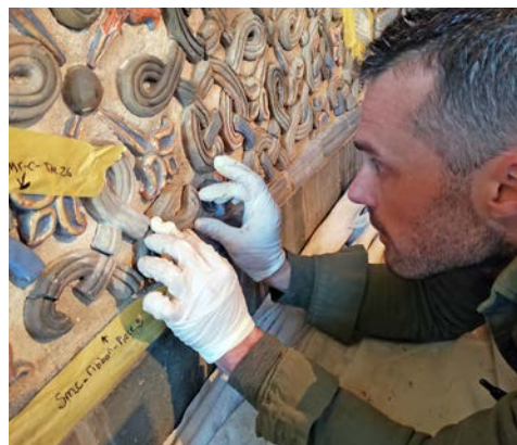
Restoration contractor Clint Flack re-attaches a tile in Fonthill's "Smoking Room."
